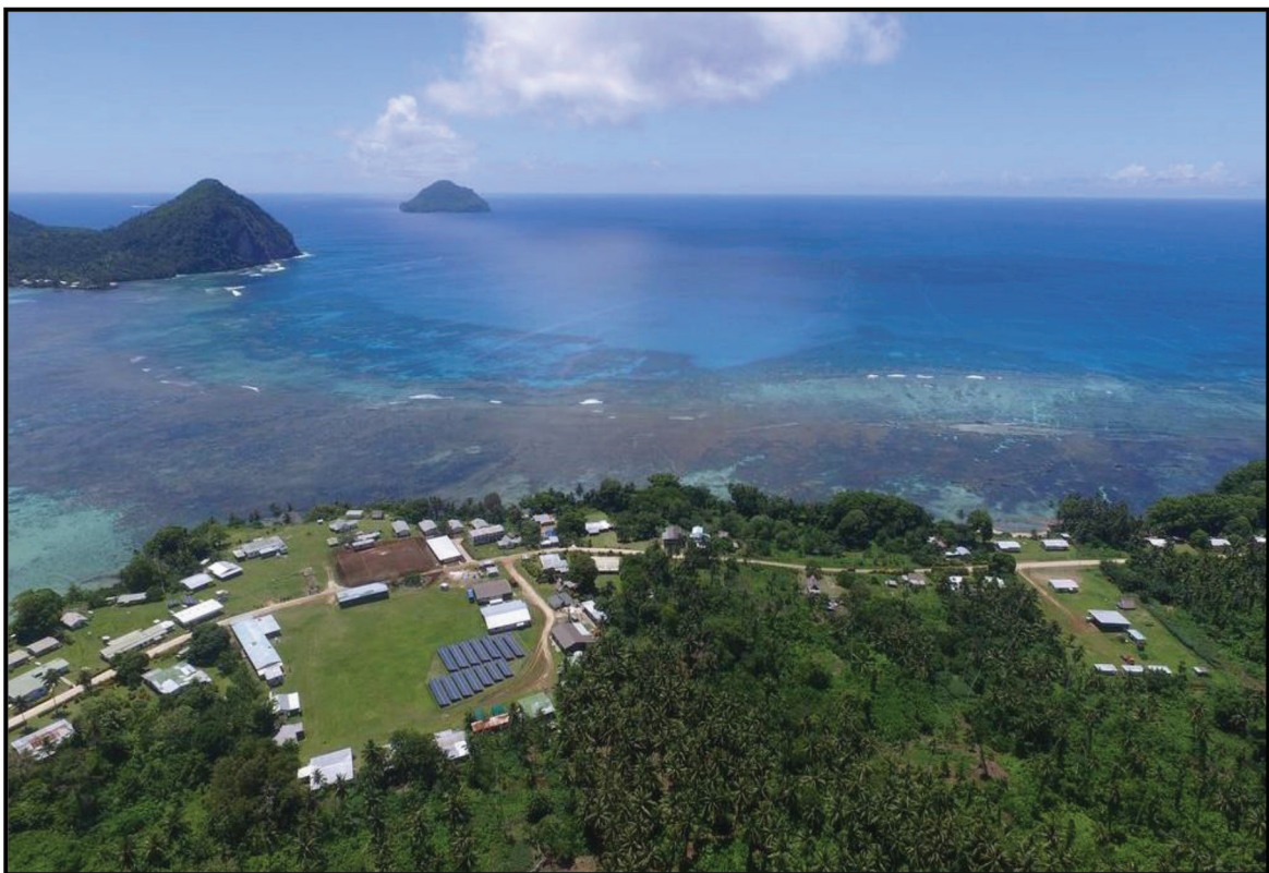
Solar Panels in Rotuma
